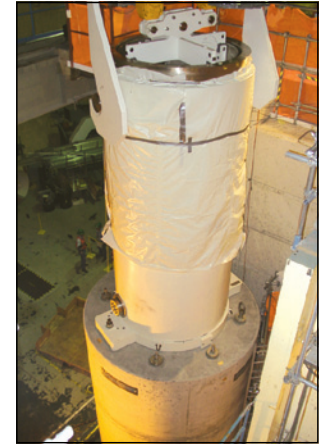
Spent Fuel Removal from Fuel Pool (L) Removal from fuel pool; (R) Inserting canister into concrete cask
